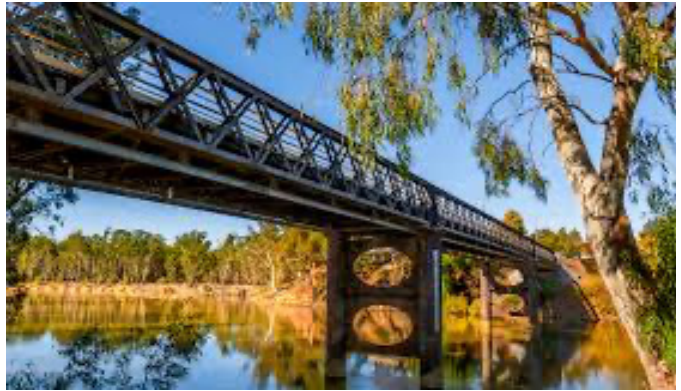
Bridge across Murray- Corowa
